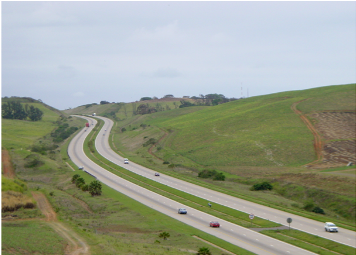
Figure 5-15: N2 North: Curvilinear alignment in a valley
