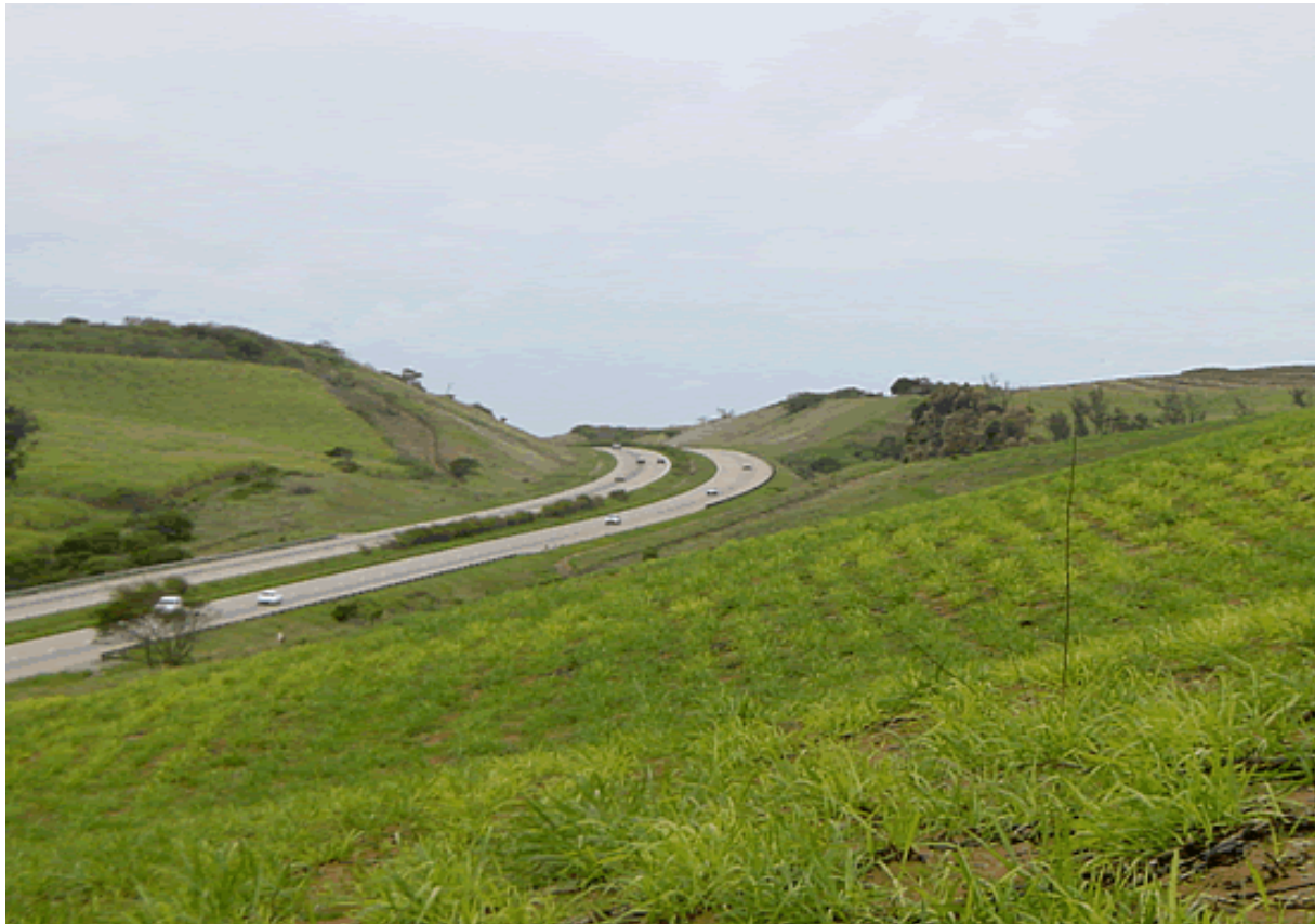
Figure 5-17: N2 - Combining horizontal and vertical alignment
