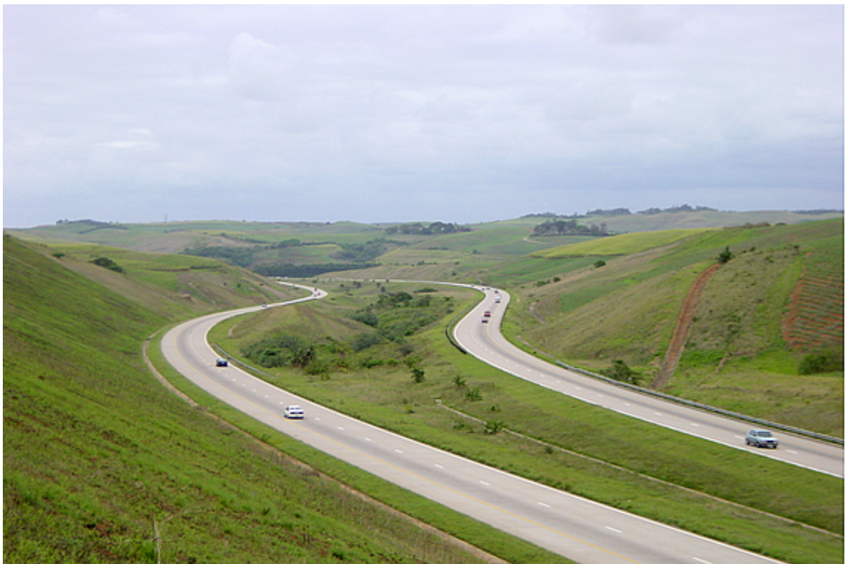
Figure 5-16: N2 North - Median widening to accommodate stream
